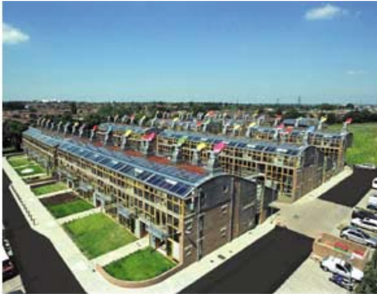
Figure 2: BedZED Ecovillage, London
